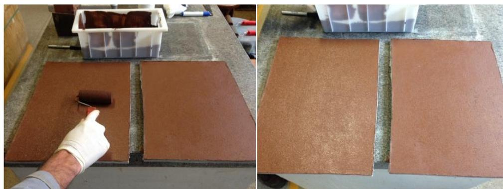
**Figura 27- PRIMEIRA DEMÃO COMPLETA DAS PLACAS PARA AMBIENTE INTERNO E EXTERNO**
